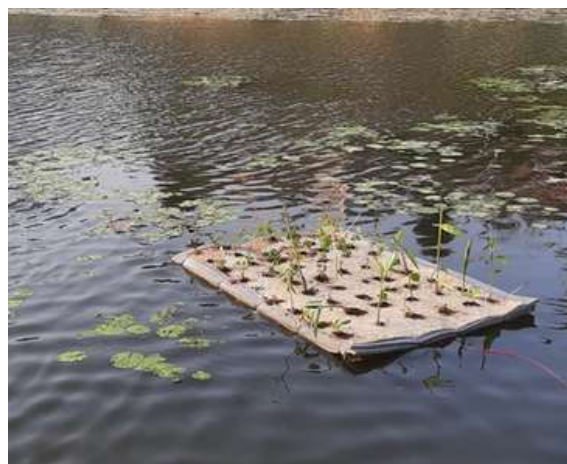
Floating Treatment Wetland System construction and installation at Nagdaha
