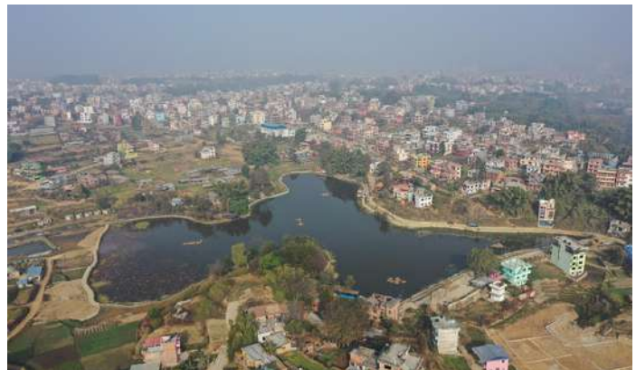
Floating Treatment Wetland System at Nagdaha from aerial view
